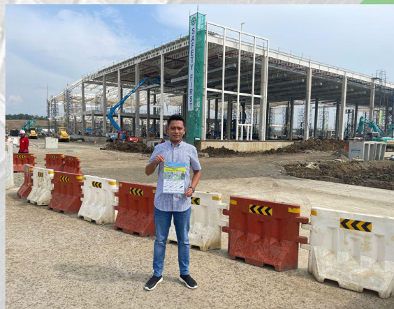
Project LG Battery Karawang
